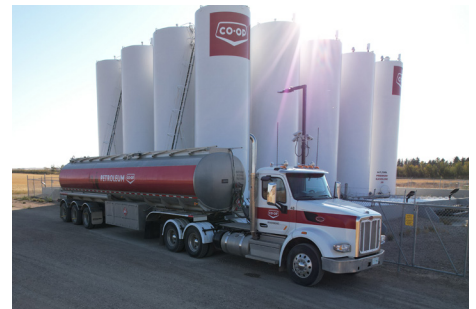
Outlook Bulk Fuel Plant, Spring 2023
